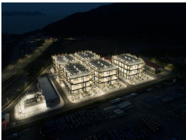
Daesan Green Energy Project 50 MW | 114 Units | South Korea
