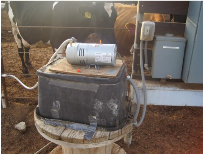
Figure 8: New air pump installation at Stockdale Dairy Digester
