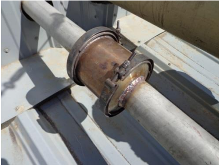
Figure 10: H-SCR catalyst
