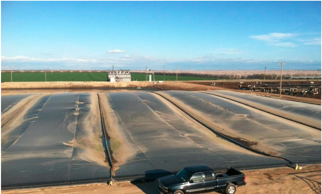
Figure 1: Covered Lagoon Digester and Engine-Generator System.
