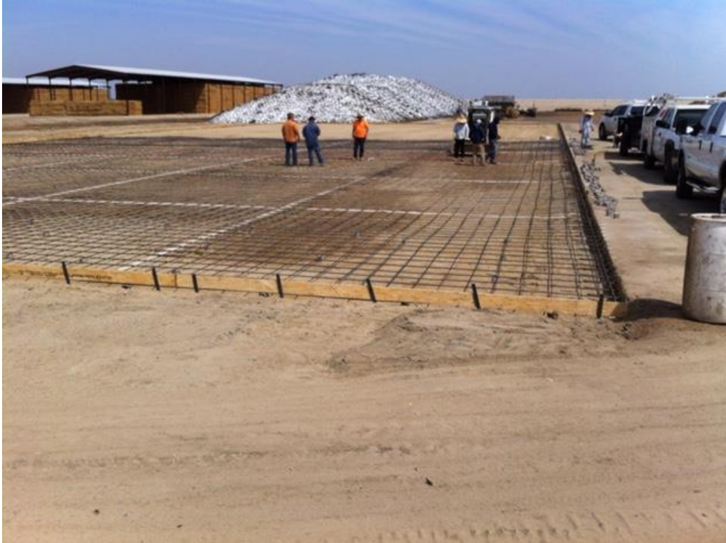
Picture 1: Preparation of the concrete slab area
