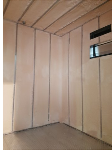
Spray foam Insulation
